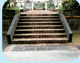
因應急降豪雨裝設雨水導水溝引導雨水排放
